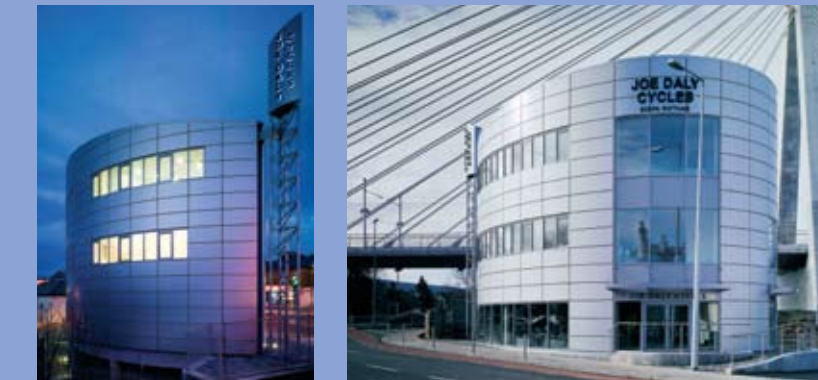
Below: Rear view of building Below Right: Entrance view from main street
